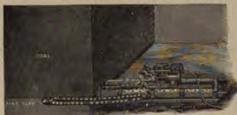
Position of Machine at Work.
